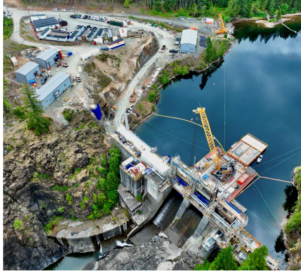
June 15: Ladore Dam and construction site.
