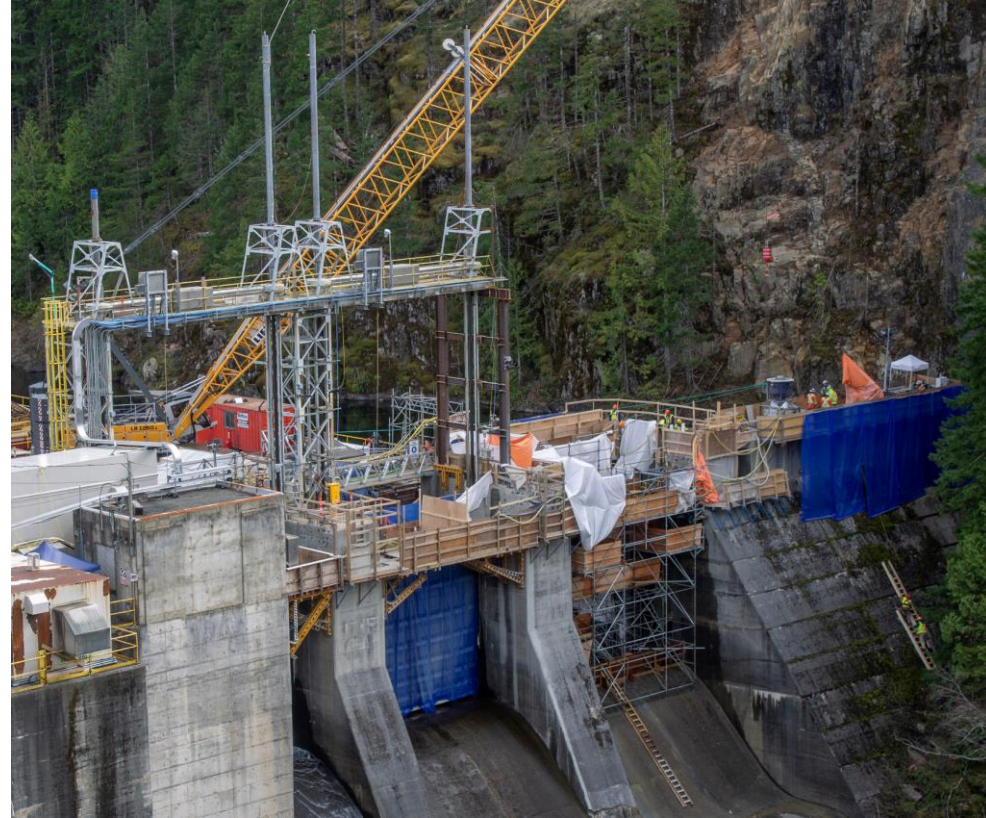
April 20: Work on the Ladore Dam spillway gates and anchor drilling.
