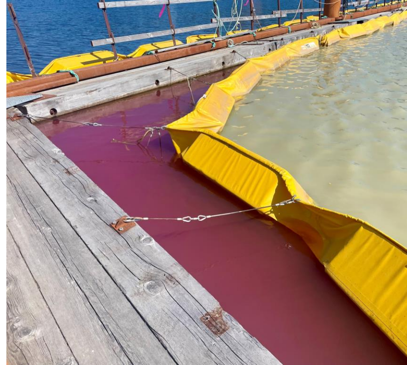
July 22 view of Rhodamine, a pink dye that is safe for the environment, placed between the two silt curtains to help find any potential turbidity leaks within the outside silt curtain. None were found.
