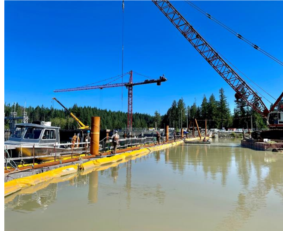
July 21 photo of crews investigating the silt curtains and possible turbidity causes, as well as the placement of geobags to better seal the outside curtain to the bottom.
