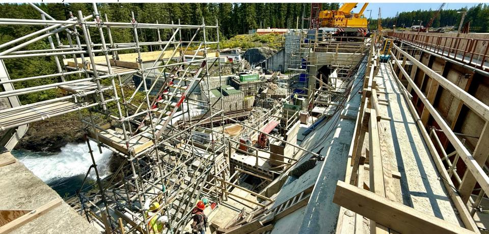
June 2 view of the drilling work to prepare for 119 steel anchors that will be installed across the length of the concrete dam.
