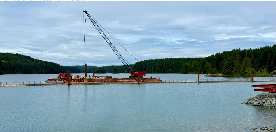
June 16 photo showing the completed placement of the downstream berm that will now go through a densification process – to compact the earthfill material.
