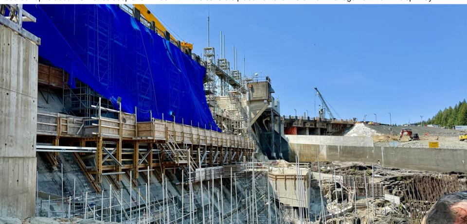
June 2 view of the removed road deck to prepare for the new overflow spillway works. A new road deck will be placed above the overflow spillway when it's complete.
