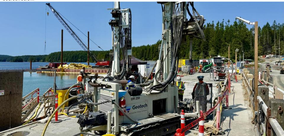
June 16 view of the anchor drilling activities from the spillway gates.
