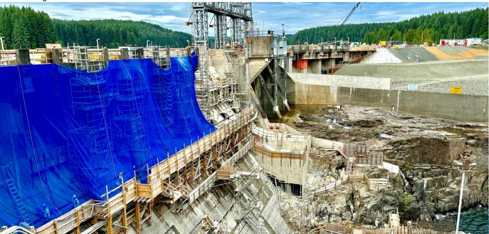
June 16 close-up view of the lower work area of the dam and all the rebar and anchors for the concrete works to manage water flow from the overflow spillway.
