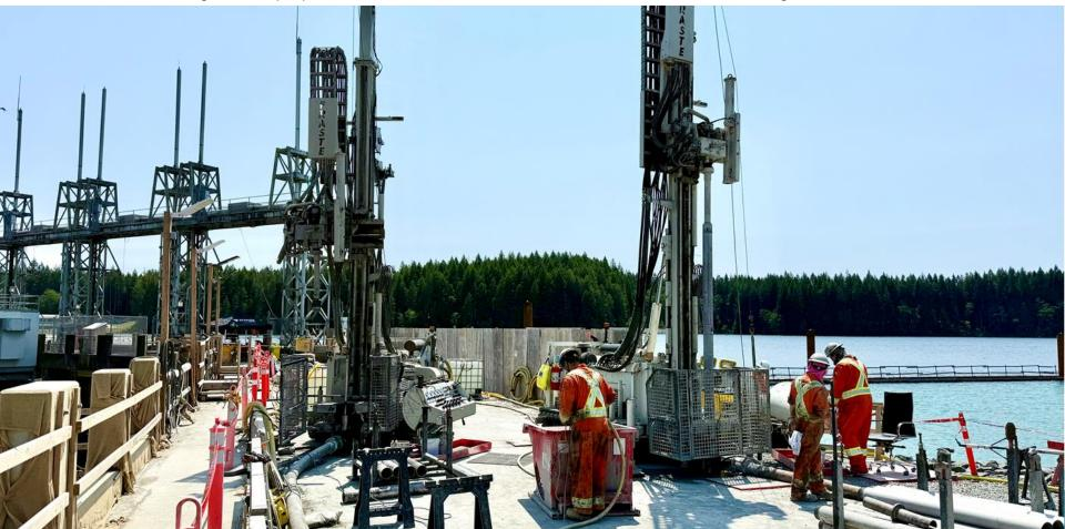
June 2 view of the drilling work. The drill holes will be up to 42 metres deep and will pass through the concrete dam and into the bedrock below.
