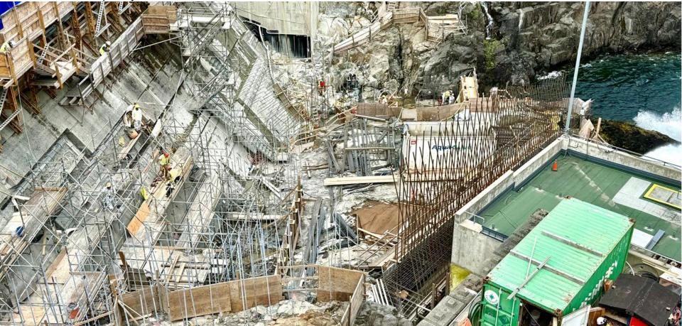
June 19 view of the downstream side of the dam and the removal of a section of the road deck for the overflow spillway.
