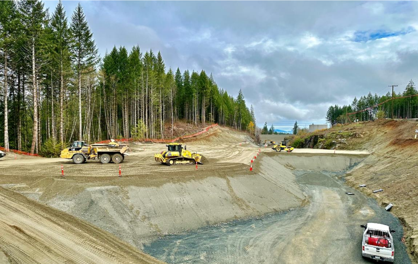
November 17 photo of the berm work progressing.
