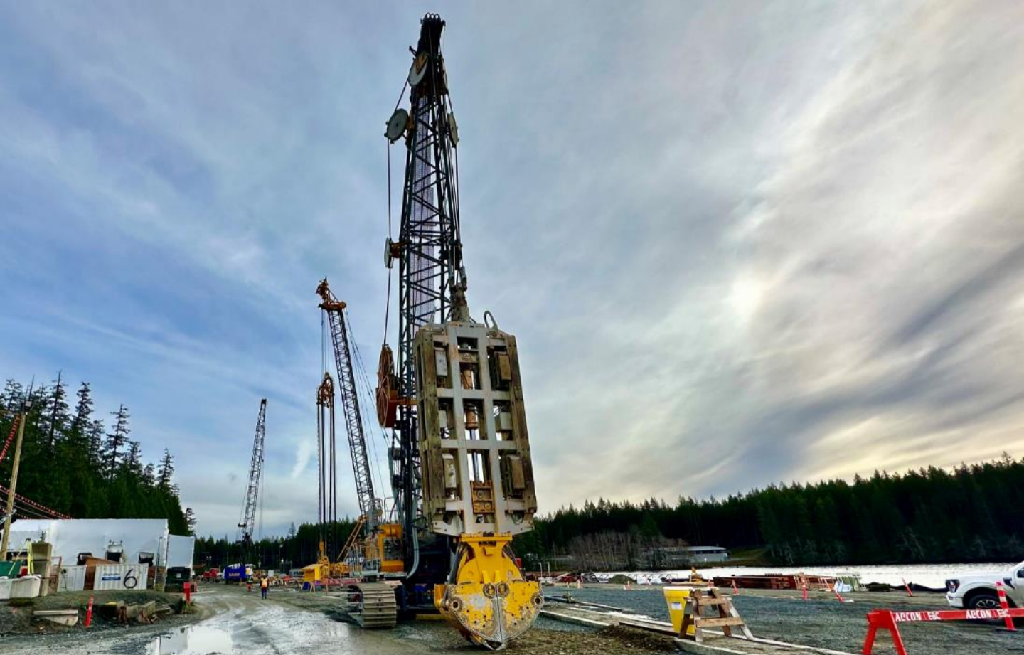
December 7 view across the dam to the work activities.
