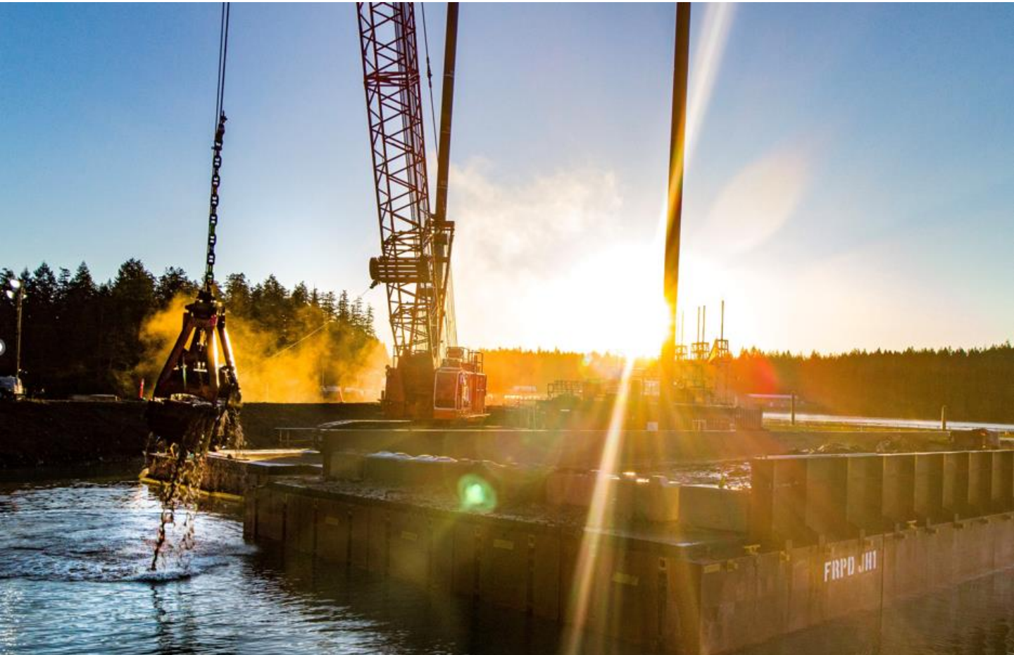
An early morning November drone photo of the barge work.
