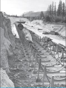
The first woodstave penstock being built in September 1947
