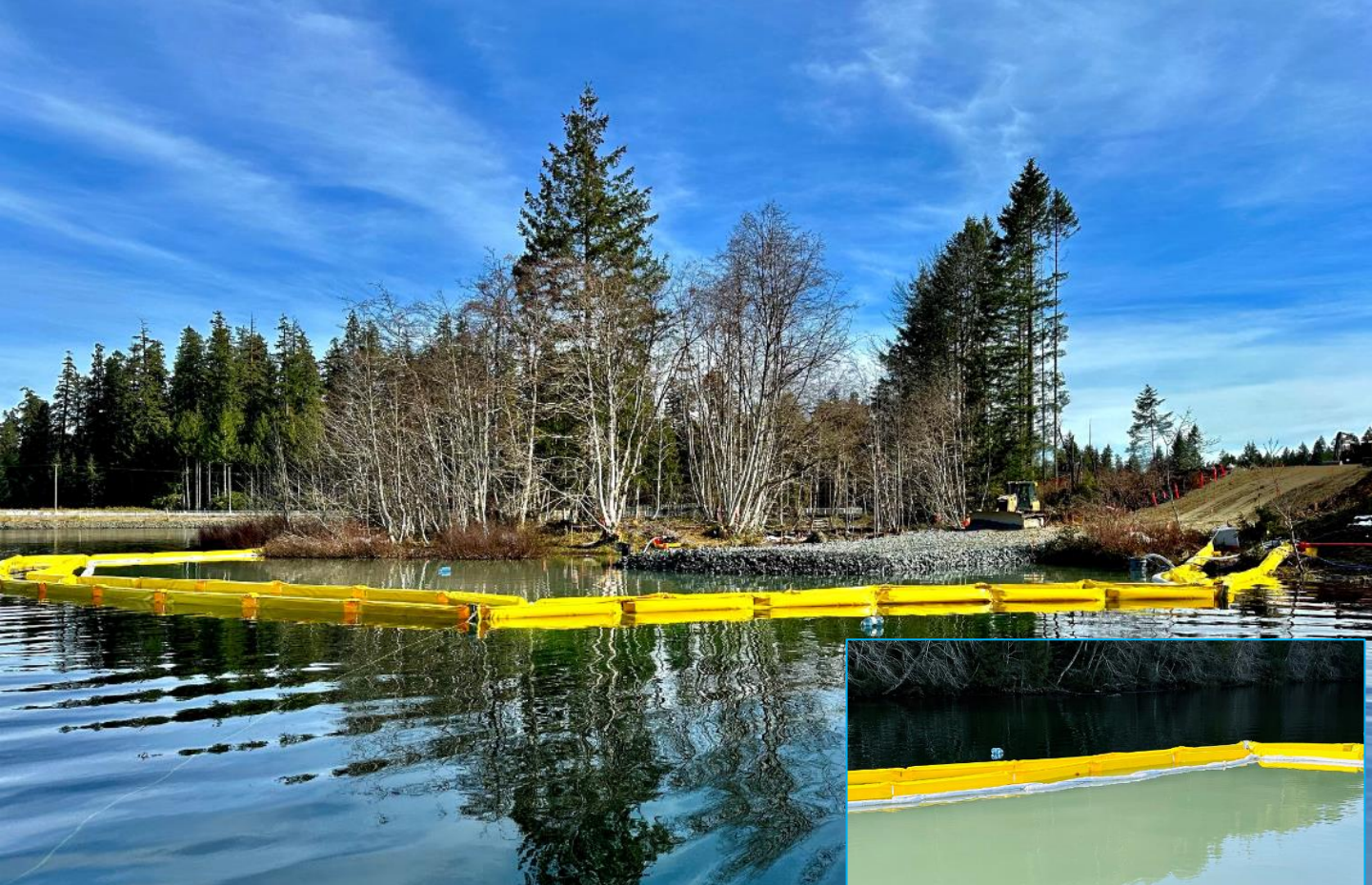
The double silt curtain around the boat ramp work zone. The insert photo shows the contained water turbidity with the rest of the reservoir being clear.
