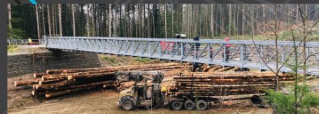
Construction activity in January 2023 beside the pedestrian crossing
