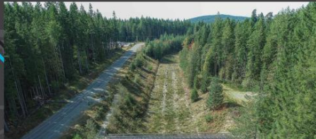
The old penstock corridor in September 2021
