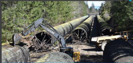
Penstock removal work in March 2019
