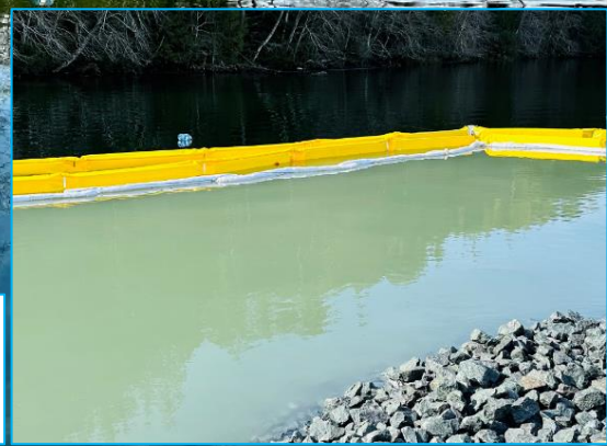
The double silt curtain around the boat ramp work zone. The insert photo shows the contained water turbidity with the rest of the reservoir being clear.
