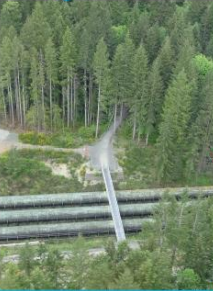
View of the pedestrian crossing over the old woodstave penstocks
