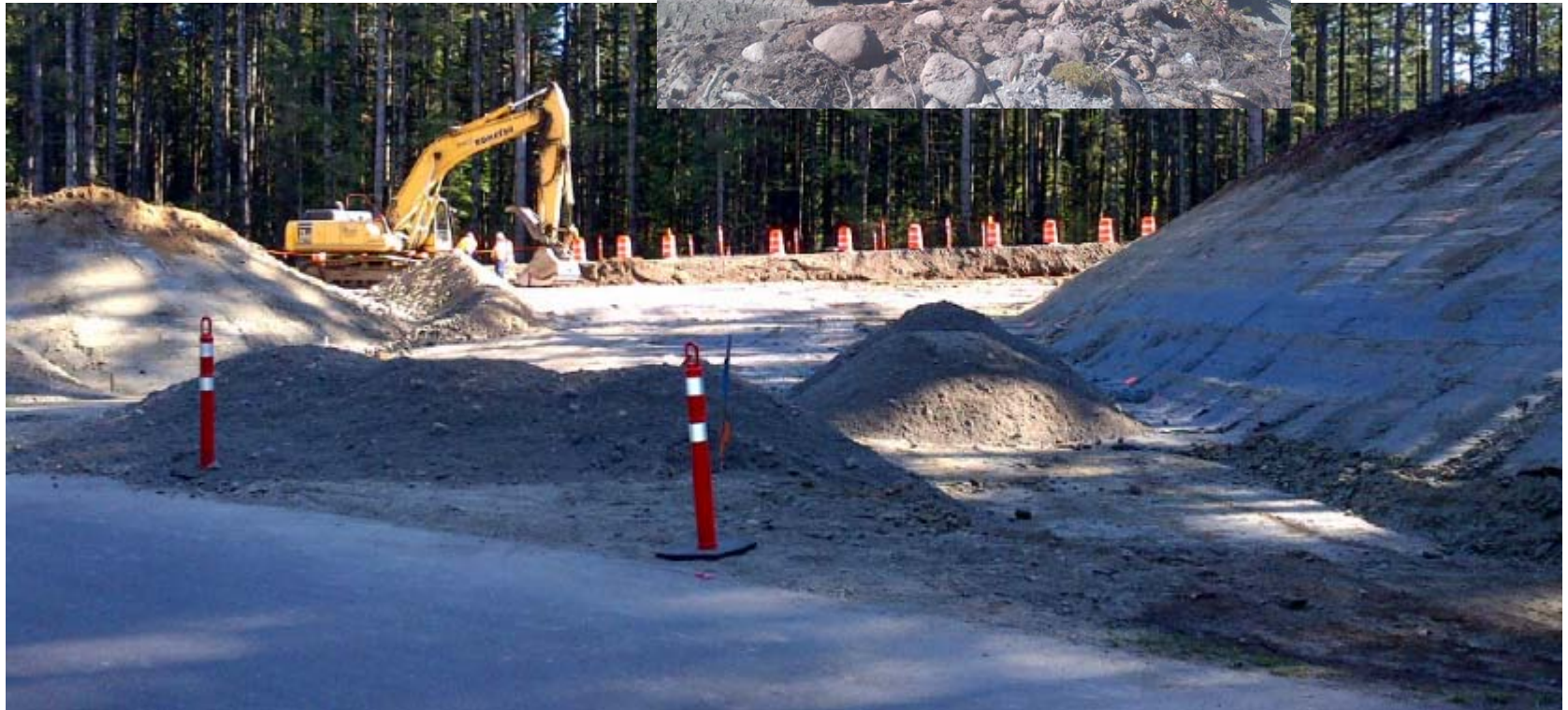
Earthworks on the future access road into John Hart.
