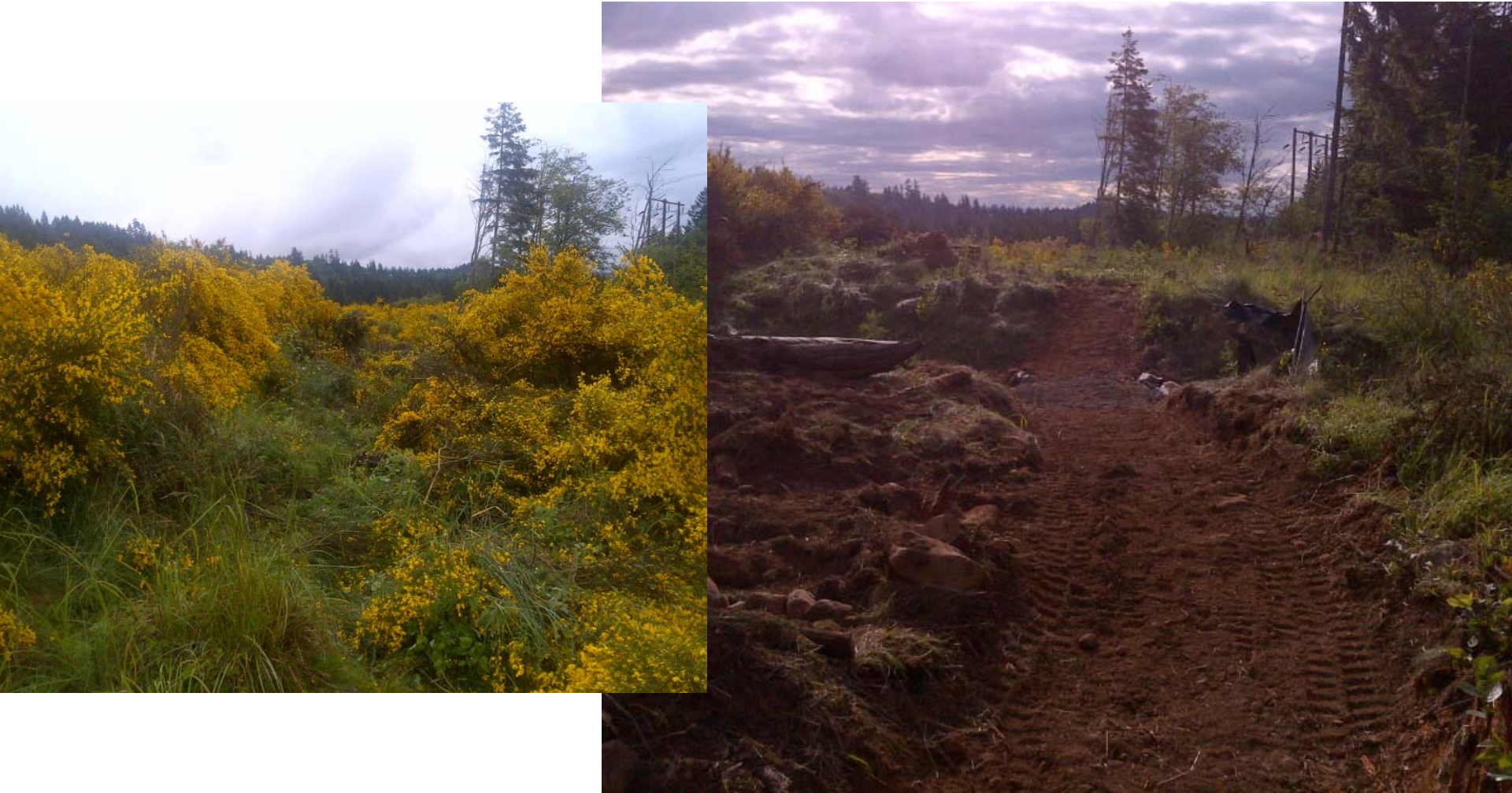
Before and after of the trail area by transmission line right-of-way.
