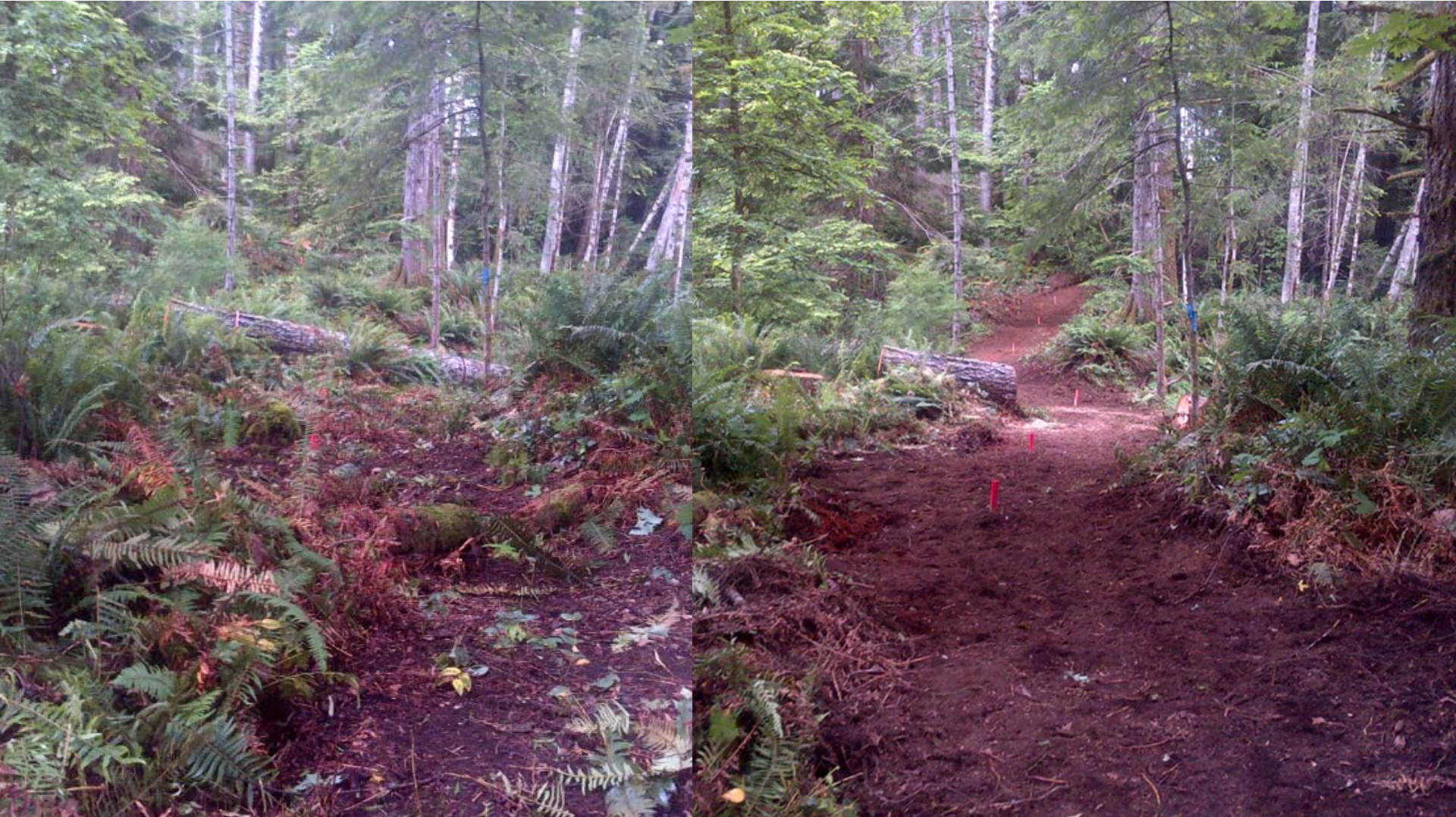
Before and after pictures along the top of the hill.
