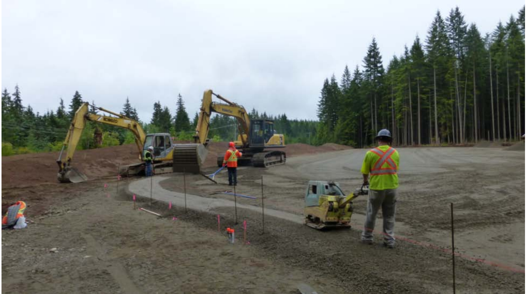
Parking lot curb preparation.
