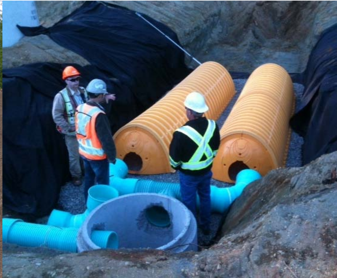
Drainage work and Stormtech chamber installation.
